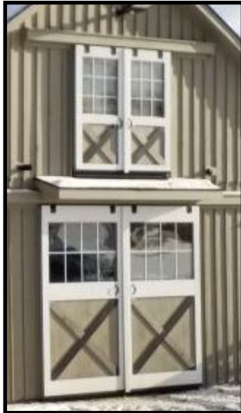
Double Sliding Doors Above Center Aisle
