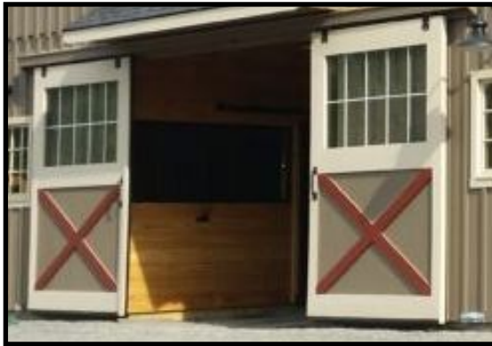
Tempered Glass In Aisle Doors
